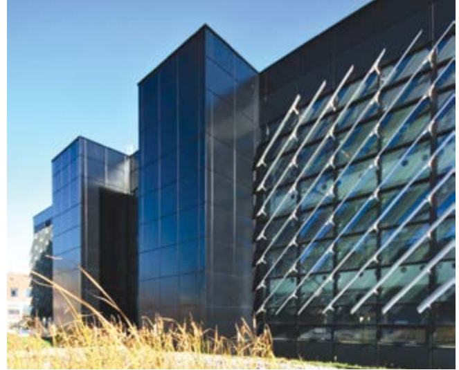
Figure 6.5 Brise-soleils en position diagonale
