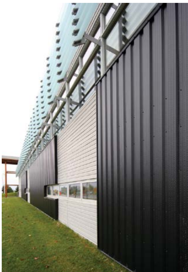
Figure 12.6 Mur solaire
