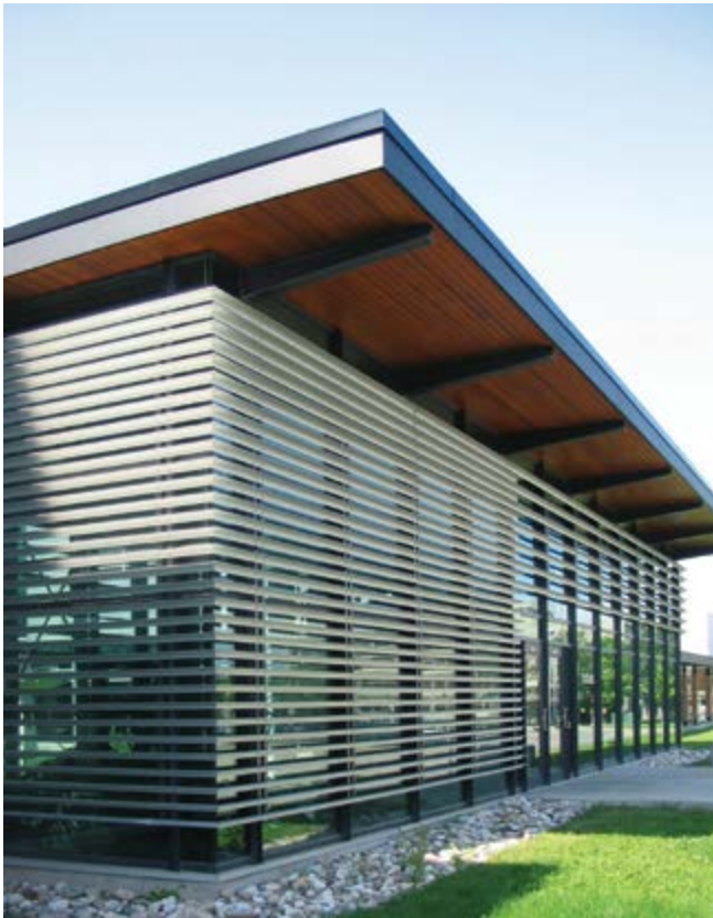
Figure 6.4 Brise-soleils en position horizontale
